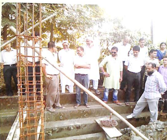
Laying foundation of new College Building
